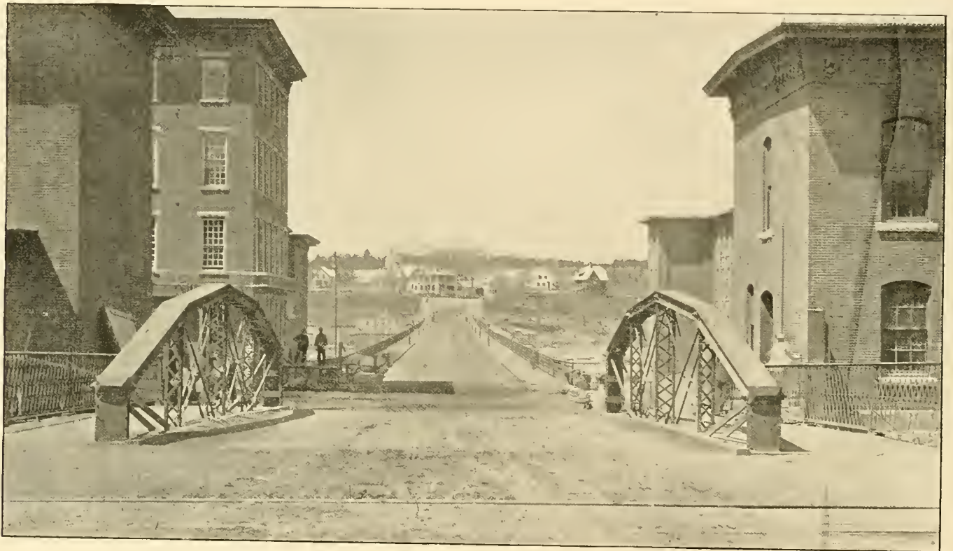
MCGREGOR BRIDGE, MANCHESTER.
